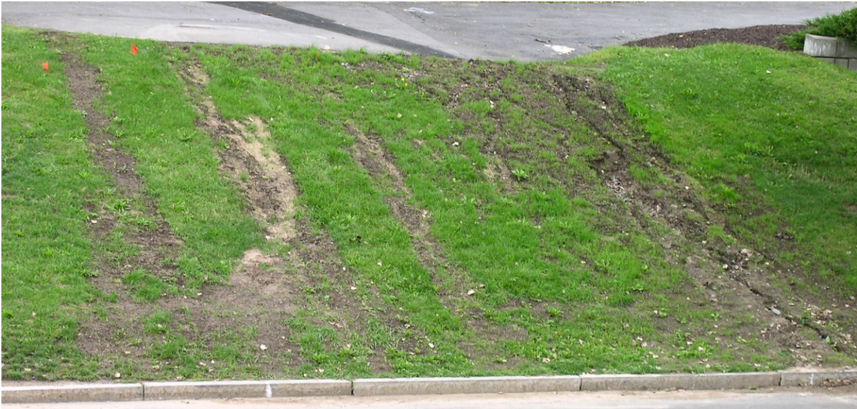
Figure 1 Rills on a roadside in central New York, USA.
