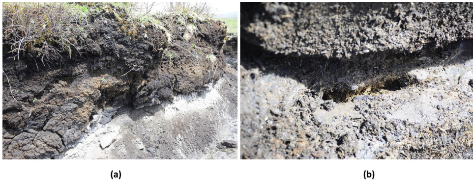
Fig. 10. Evidence of cracks and small holes near or at the bottom of the peat layer. (a) Cracks around the peat bottom; (b) Small holes at the peat bottom.
